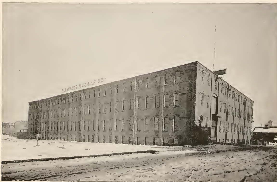
BUILDING OF THE S. A. WOODS MACHINE COMPANY.
